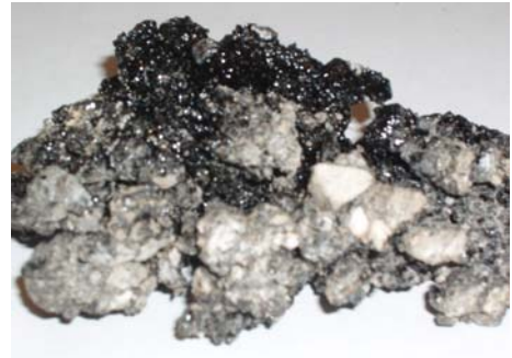
Figure 6: Clogged Layer of Porous Asphalt
