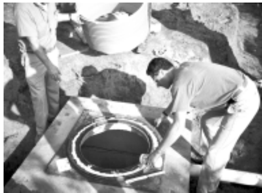
Your contractor should install access risers to grade on your septic tank.
