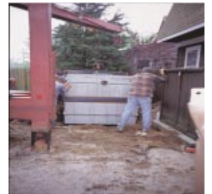
Installation of concrete septic tank.
