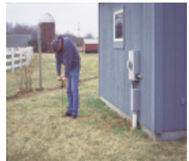
Locate the septic tank by probing with a metal rod. Be sure to avoid underground electric lines. Do not probe where there may be underground electric lines.
