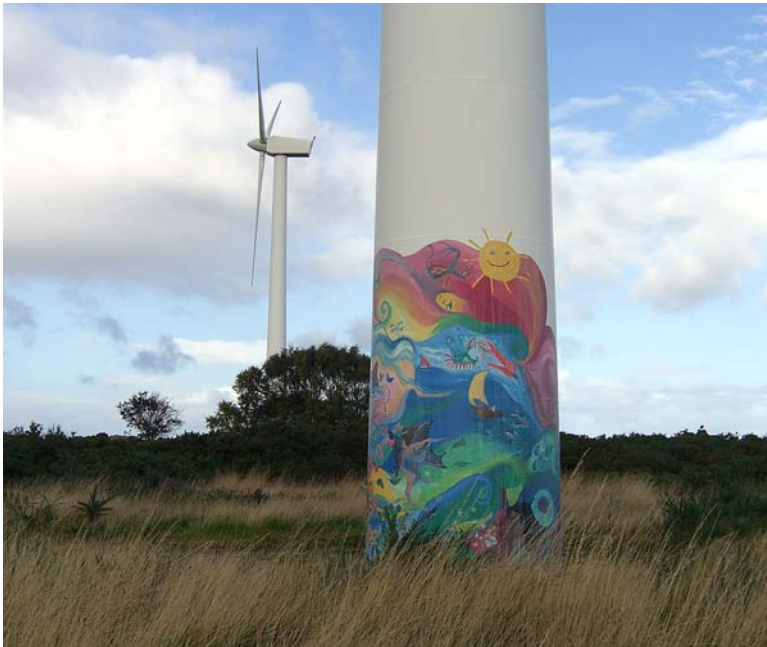
Painted Tower at the Findhorn Eco-village Wind Farm, Scotland
