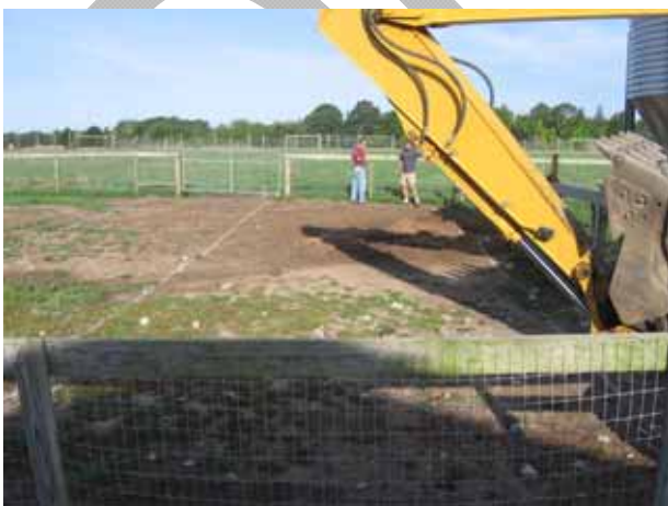
Areas where livestock yard will be retrofitted are outlined in white
