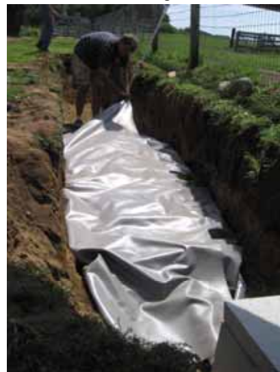
Once filled with woodchips, the bioreactor is backfilled with native soils.
