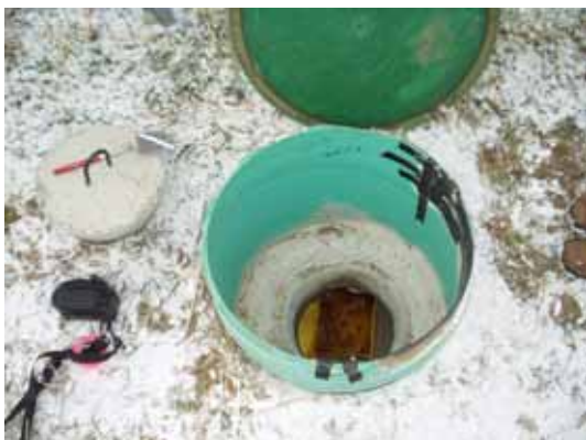
Tipping bucket and groundwater sampling port upgradient of wood chip bioreactor at URI Peckham Farm
