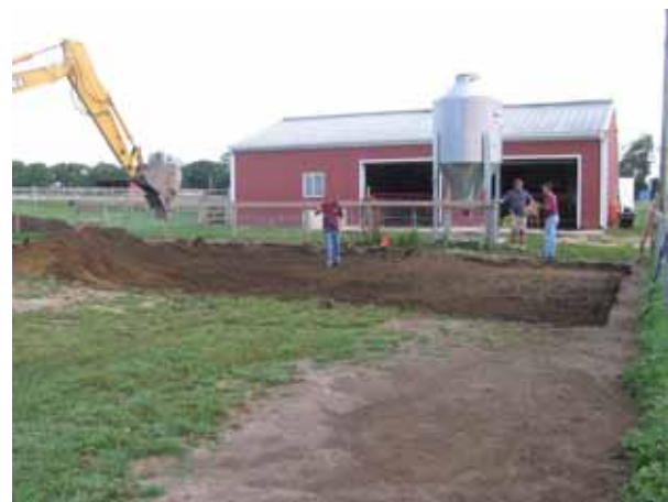
Excavation of area to be retrofitted
