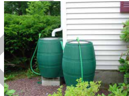
Rainbarrels provide rainwater storage for later use (CRMC and RIDEM, 2009)
