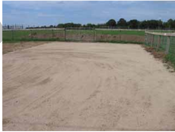
The final test infiltrative areas after both systems are installed.
