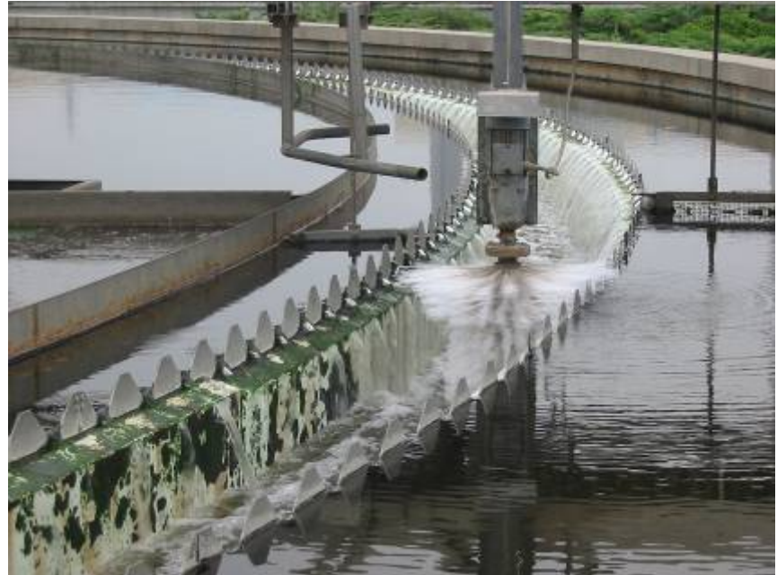
Gaobedian Waste Treatment Plant
